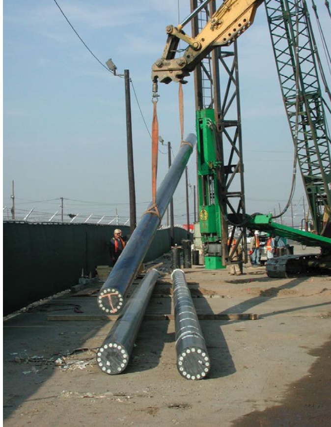
Plastic piling at Iskander's research site.
